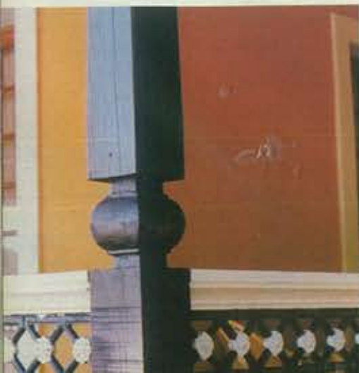
BELOW: The carpentry work was exquisitely crafted by traditional craftsmen. The detailing is very typical and has been done in specially treated sal wood.
