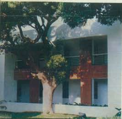
BELOW: In attempting to be one with nature a new dimension has been given to conventional corridors.
