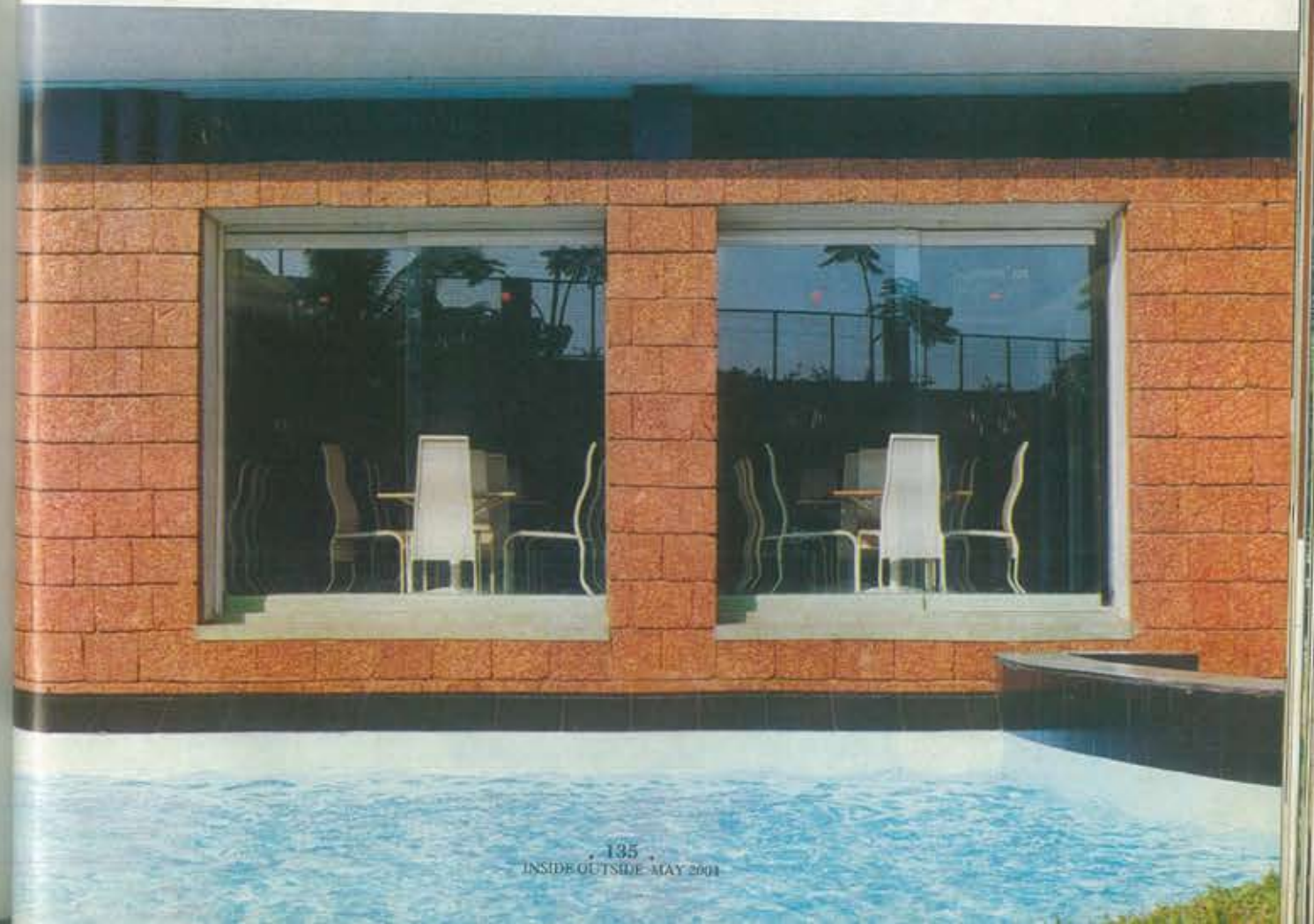
BELOW: The clear glass panes of the canteen give diners a view of the tranquil, cool blue water body, in harmonious contrast to the rough texture and opacity of exposed laterite walls.
