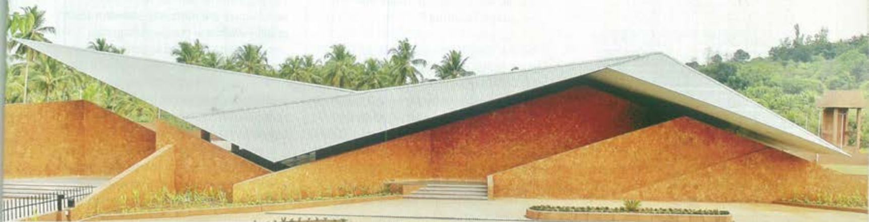
† The scale, sensitivity to its context and composition are co-mingled and reshaped to refine a new architectural language.
