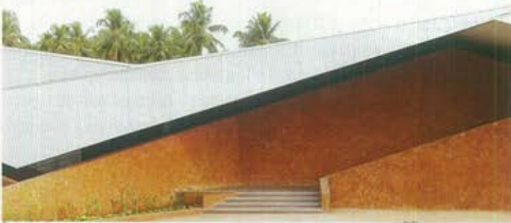
The exposed laterite walls, defining the spaces, provide a sense of direction to the visitor.
