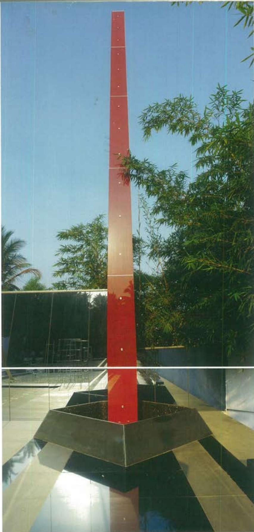
† The composite structure of the tower is a framework with M S at the core, clad with two layers of toughened glass in a carefully chosen shade of red.
