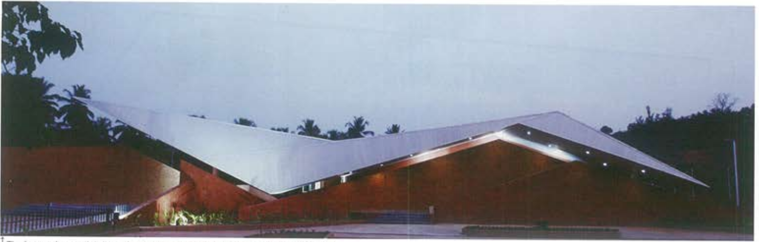
† The inconspicuous lighting enhances the roof's expression as a stroke of lighting.
