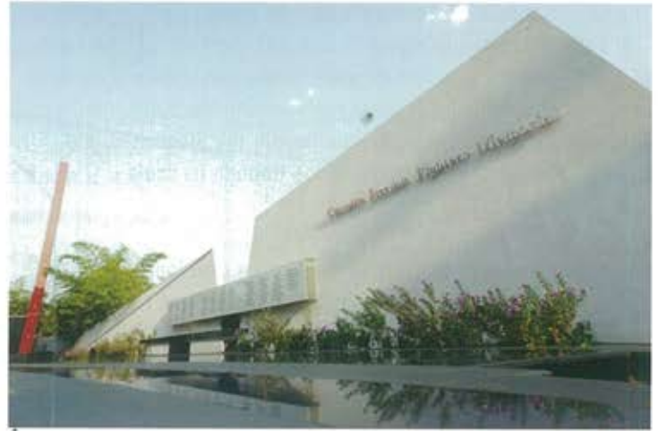
↑ The white angled walls depict the repressing Portuguese regime while the black granite flooring reference the suppressed dark-skinned native Goans.
