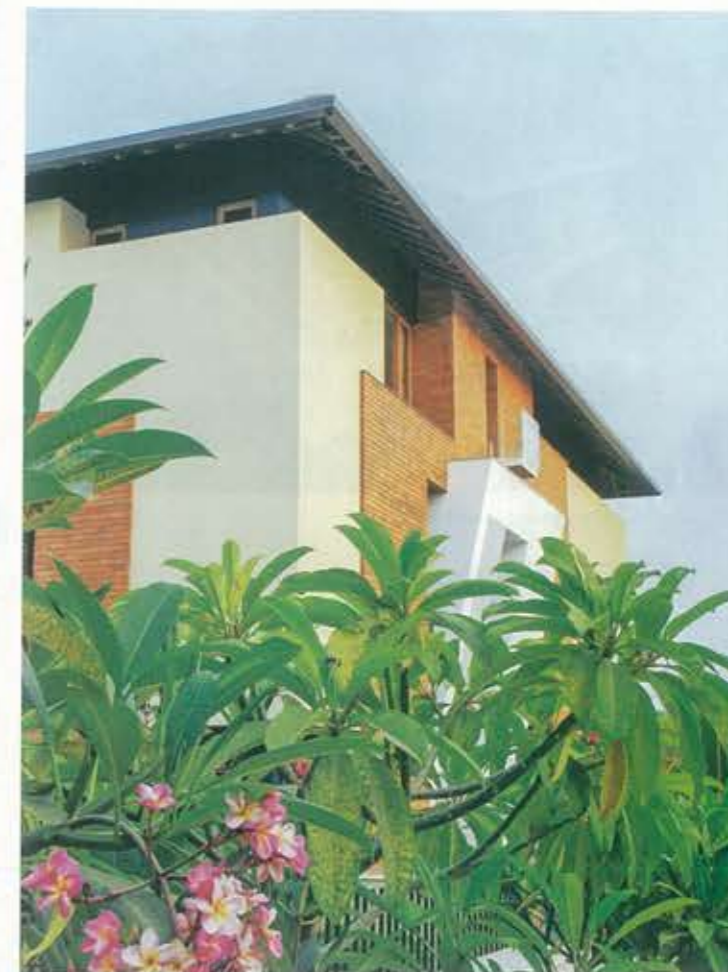
The roof complementing the form of the building
